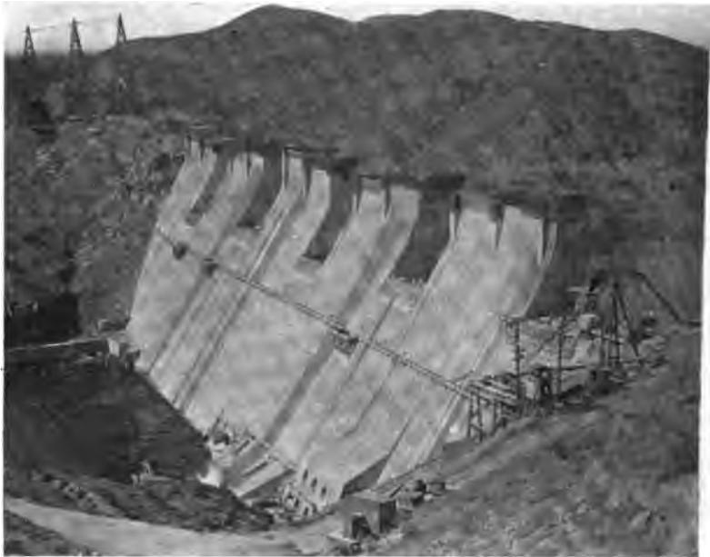
FIG. 222.—Elephant Butte Dam, showing Construction in Alternate Columns.
